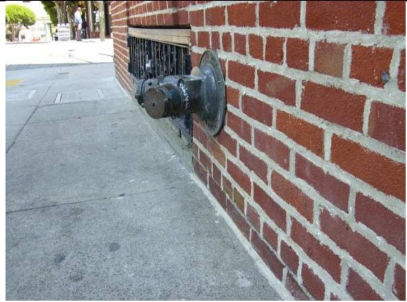
Standpipe A Side View
