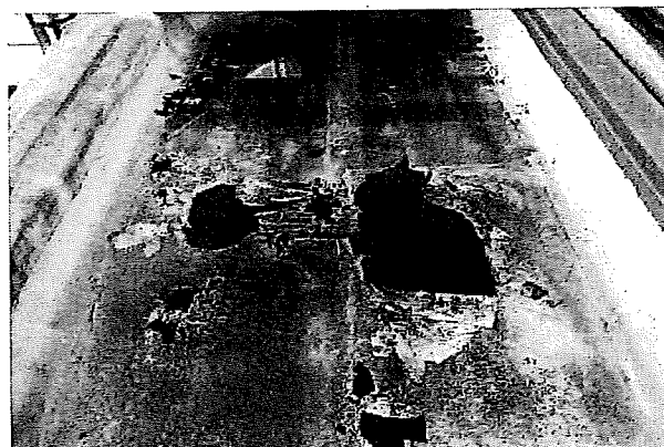
PHOTO #30: Roof Covering
