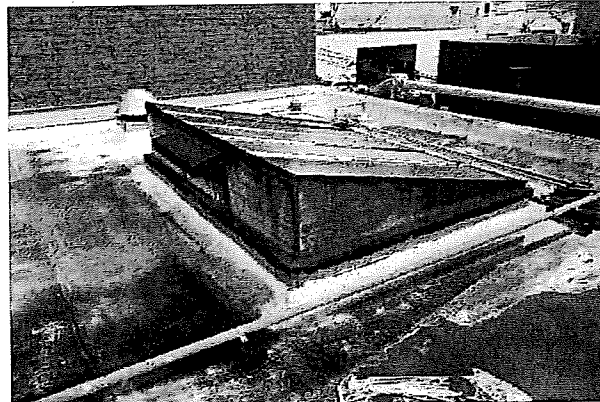
PHOTO #26: Roof Covering
