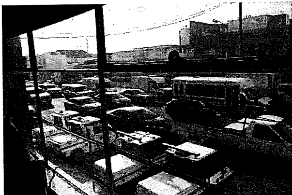
PHOTO #5: Steel frame window
